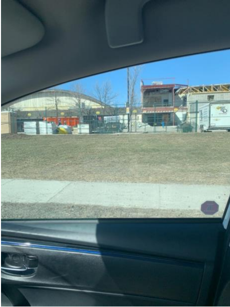
Figure 1 Looking north - the office is gone!
