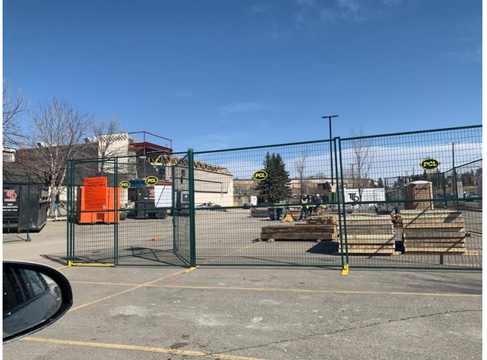
Figure 2 Looking east into the JC parking lot
